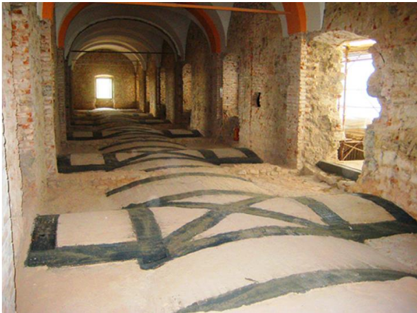
Figure 12. reinforcing system with FRP, ex-monastery in Bergamo (Italy), (project by Building Improving S.r.L)
