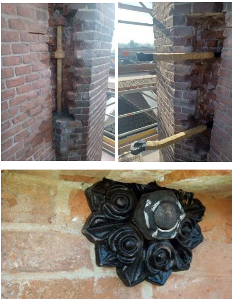
Figure 4. concealed new anchoring and anchor plate at the extrados – all historically restored techniques
