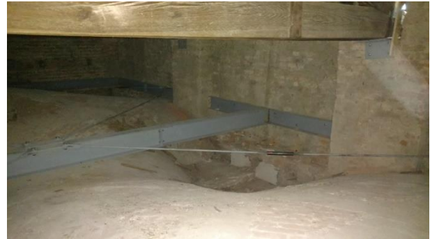
Figure 10. Steel diaphragm above the vaults (Palazzo Botta Pavia – project by Studio Calvi)
