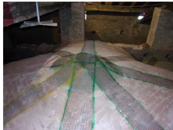
Figure 11. Application of basalt fibre mesh and covering with NHL mortar, Santa Monica – Cremona (project by Studio Calvi)
